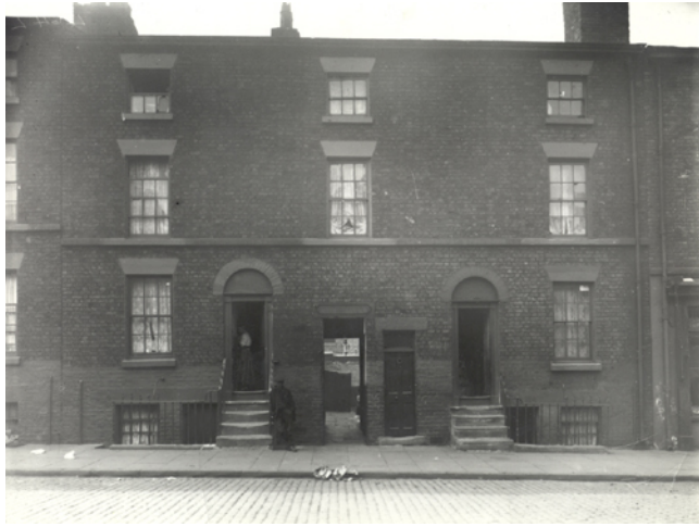
Figure 4.8: A typical entrance to a court, similar to the house where the Canevali's lived in 1841. Entrance to No.26 Court, Burlington Street, 1925
